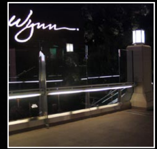
Pedestrian Bridge, Las Vegas, NV
